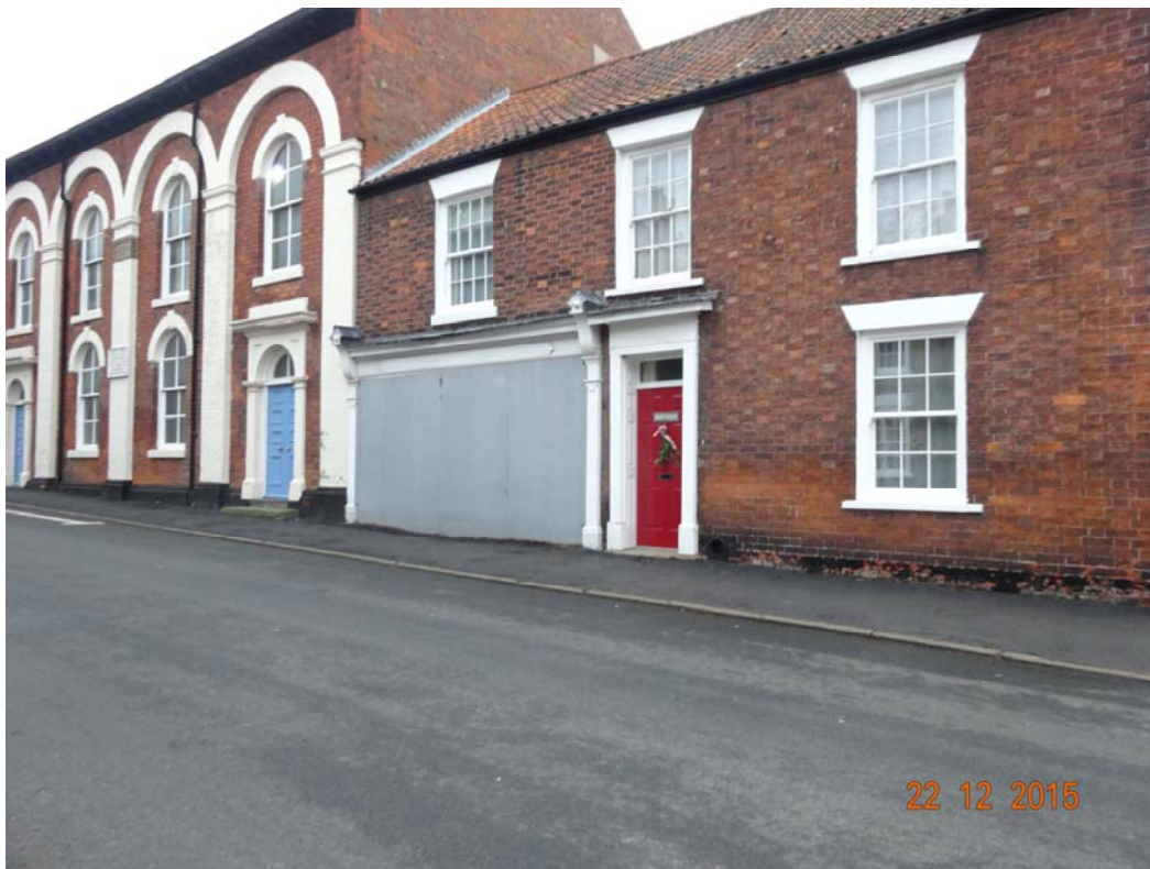
Existing Elevation – Boarded up
