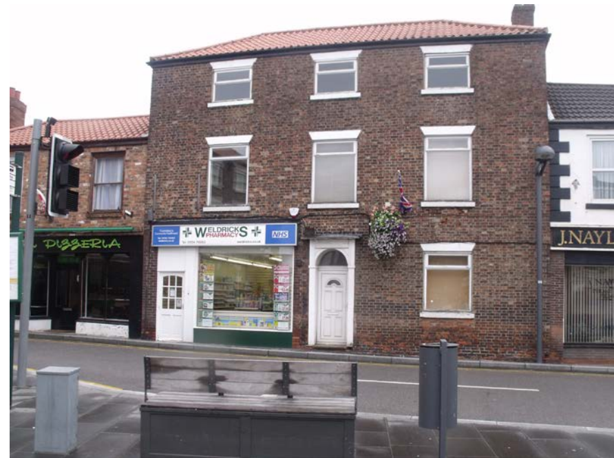
Figure 2: This modern shop front has no visual relationship with the upper floors.
