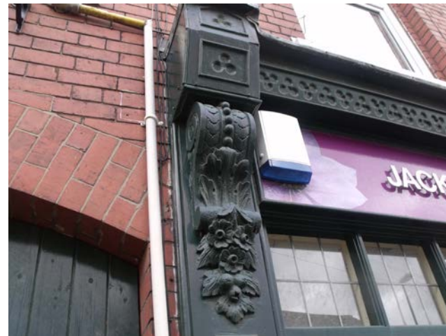
Figure 7: Ornate Victorian console bracket
